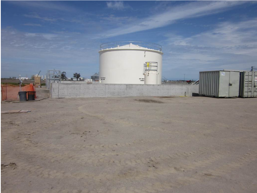
Photo 1: Saltwater storage tank at the Remote Well Pad site. Tank has been painted and containment dike around the perimeter has been completed.
