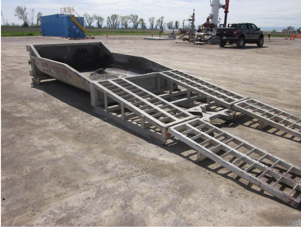
Photo 3: Concrete washout provided at the Remote Well Pad site.
